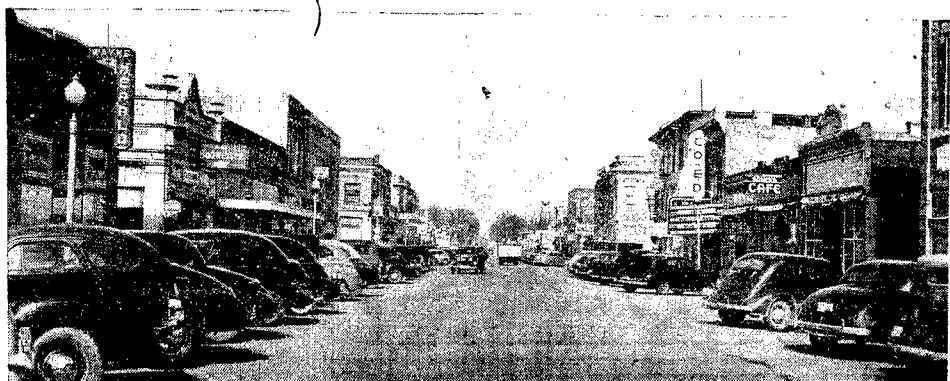
EXAMPLE OF WAYNE'S PAVING.—HAS INSURED CLEANLINESS AND CONVENIENCE
